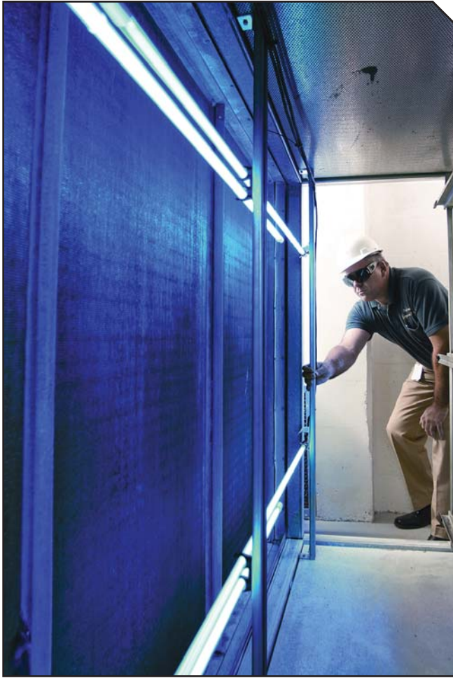
FIGURE 3. Note the person checking the installation is wearing protective eyewear, and that the safety interlock for turning off the lights when the access door is open has been overridden. (Image courtesy of UV Resources.)
