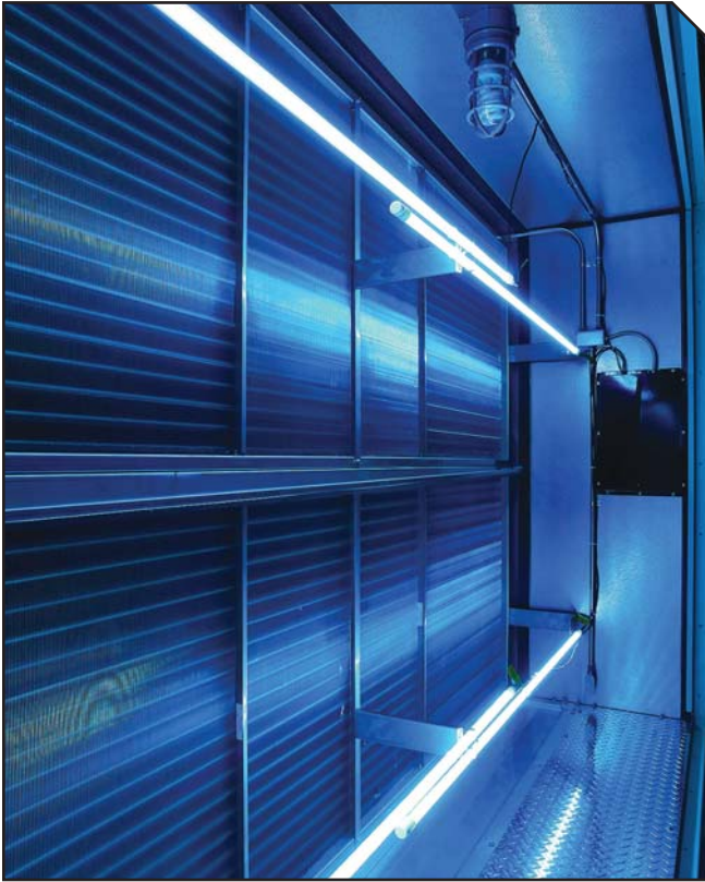
FIGURE 1. Overlapping lamps enables installation of uniform lengths, which makes re-lamping easier. (Image courtesy of UV Resources.)
